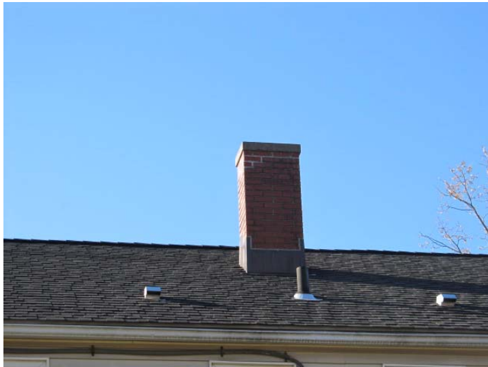
Newer composite asphalt shingles typical on all buildings
