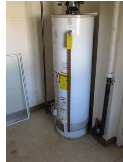
Typical unit-level natural gas-fired domestic hot water tank
