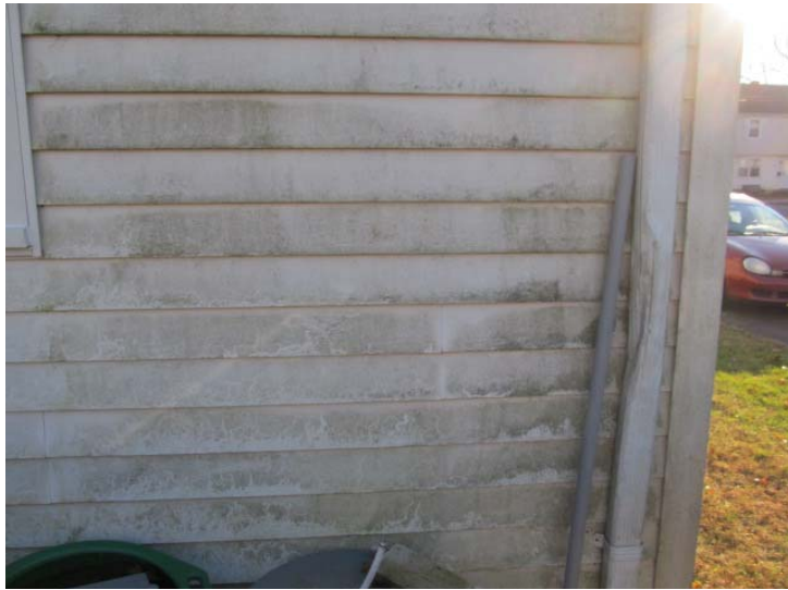
Dirt/organic growth on surface of vinyl siding is widespread throughout the development
