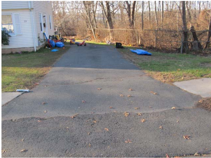
Typical asphalt-paved driveway – Surfaces in fair to good condition at the present time
