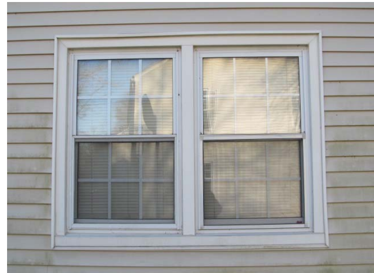
Typical aluminum-framed windows – Replace concurrent with vinyl siding in future
