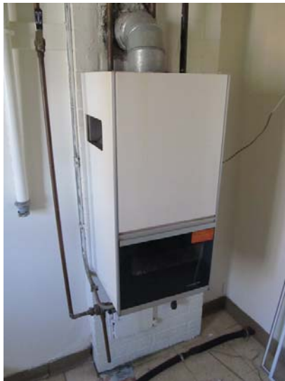
Typical wall-mounted, gas-fired boiler for unit space heating – Equipment is obsolete and repair/maintenance parts are difficult to source
