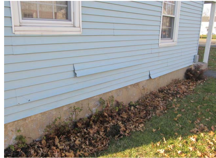
Isolated loose seams, impact damage, and faded colors also evident at vinyl siding
